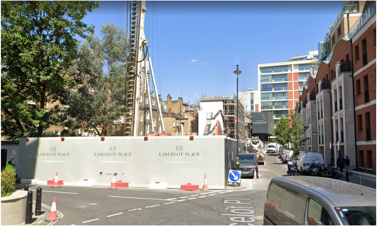
View of Application Site
